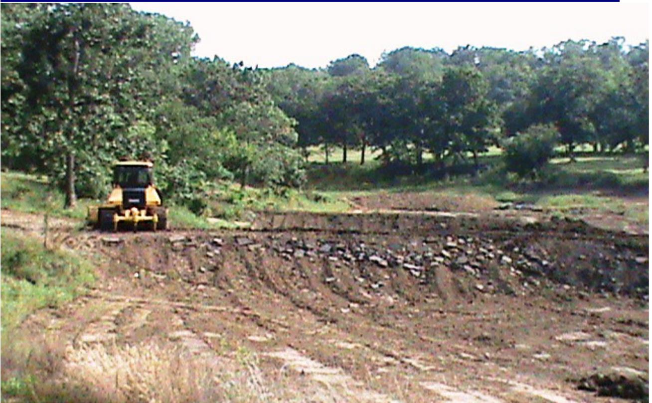
The City has completed the fishing piers, including placing riprap along the front side. A total of 6 piers have been constructed. These will double the available shoreline for angling while increasing the average water depth.
