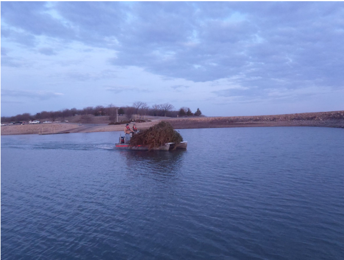
CORPS of Engineers transports cedar tree brush pile to create deep water fish habitat at Clinton Reservoir
