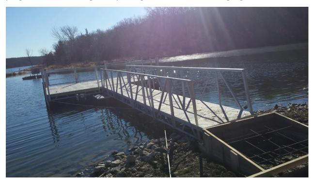
The new Mound City Lake dock. At the time of the picture the final concrete pad had yet to be poured because of the cold weather. But the City crew did a great job on this and it is finished and ready for customers. Notice we used concrete fiber walk way that is very stable, and maintenance free.
