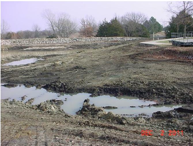
Pond depth restored, shoreline access renewed.
