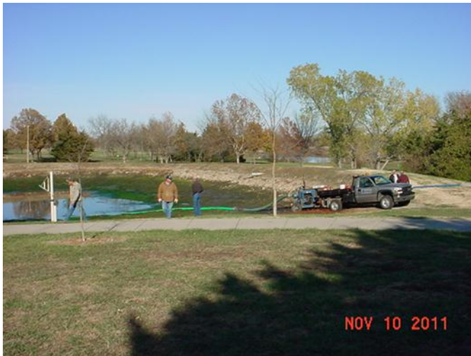
Pumping the pond.
