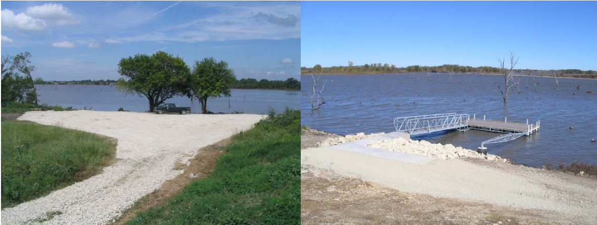
Enhanced access south of the NE 70th Street bridge.
