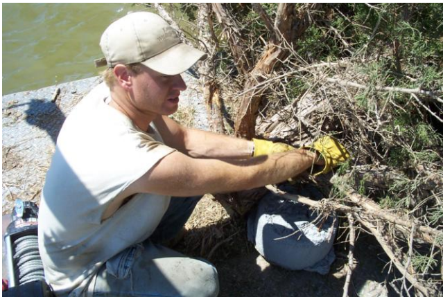
Brian wiring anchors to a tree
