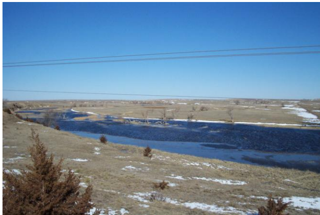
Release water flooding the previously dry Smoky Hill River 5 miles east of Cedar Bluff dam
