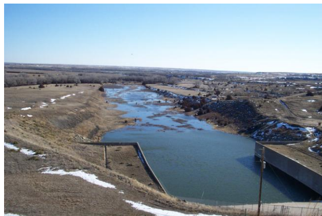
Release water backing up into the stilling basin below the emergency spillway
