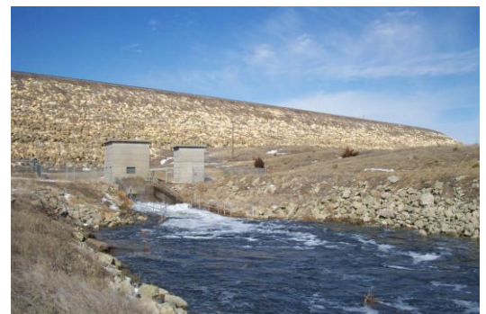
Releasing 250 cfs from the control house below the dam
