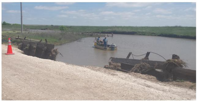
Damage on the road on the west end of HorseThief Reservoir from high water flow.
