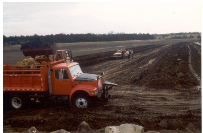
Bottom of Lyon SFL during renovation 2001.
