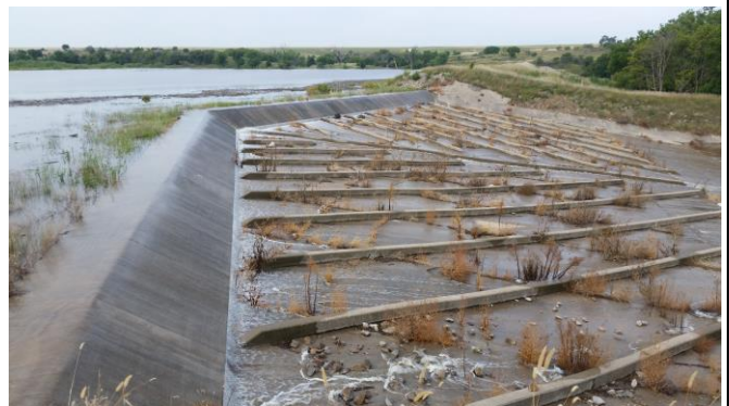
*Rooks State Fishing Lake with water going over spillway
