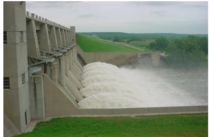
Fall River Reservoir Dam Sluice Gates Open
