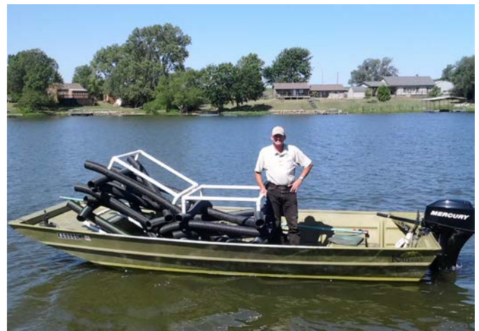
PVC fish habitat cubes installation
