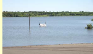
Milford Reservoir 2010 flooding
