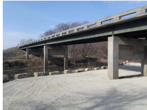
New parking area beneath the Neosho River bridge.
