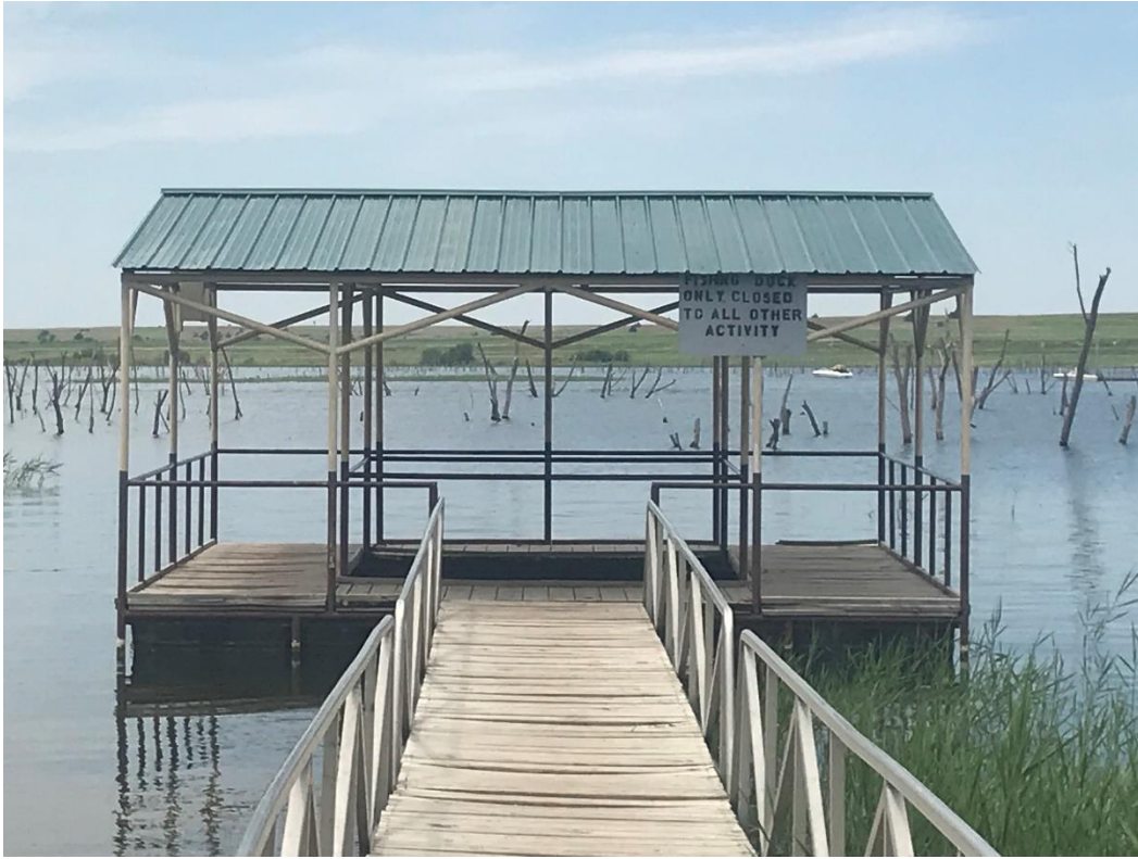
Cedar Bluff fishing dock with new, metal roof
